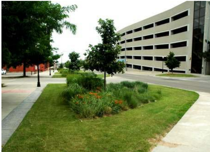
Figure 4-6 Sidewalk Median in Topeka, KS Provides Pervious Area
