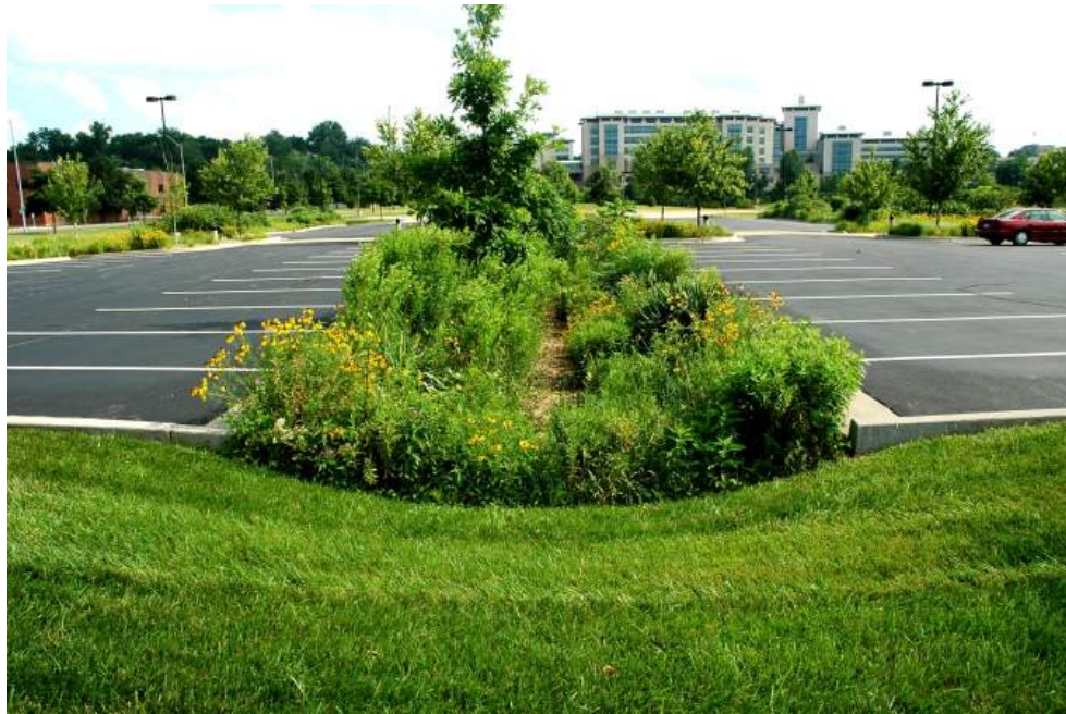
Figure 4-13 Vegetated Swale Guides Runoff From Surrounding Parking Lots Into Bioretention Cell Kansas City, MO (Source: CDM)
