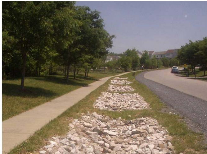
Figure 4-19 Surface View of an Infiltration Trench (Photo: MARC, 2008)
