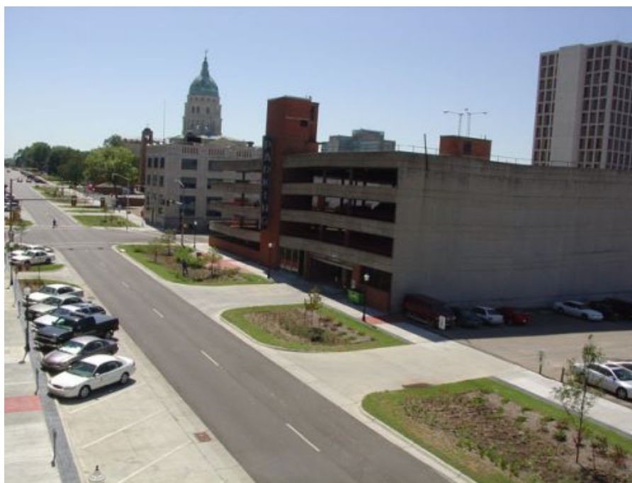
Figure 4-9 Series of Bioretention Cells on Jackson Street, Topeka, Kansas (Source: GreenTopeka.org)
