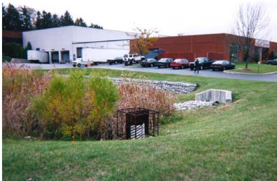
Figure 4-22 Extended Dry Detention Basin Located at an Industrial Location
