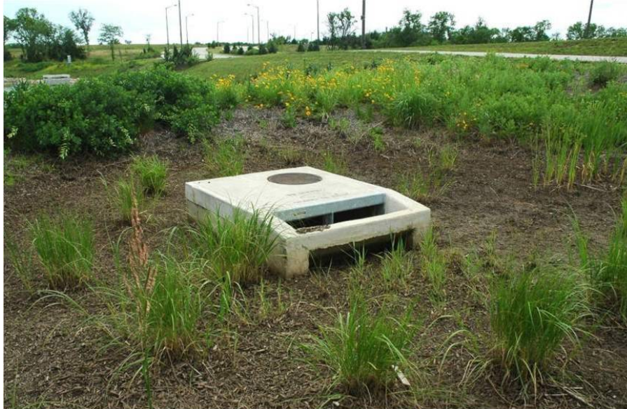
Figure 4-12 Mize Lake, Lenexa, Kansas Bioretention High Flow Structure
