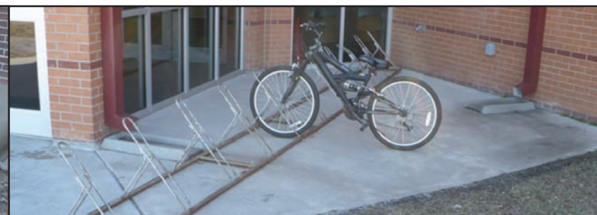
Figure 3.5 - Grid Type Bicycle Rack at Chisolm Middle School (Poor Design)
