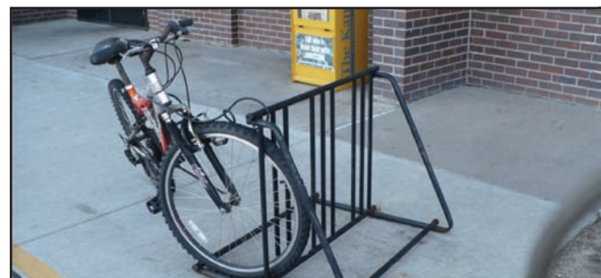
Figure 3.4 - Grid Type Bicycle Rack at the Mid-Town Towers (Poor Design)
