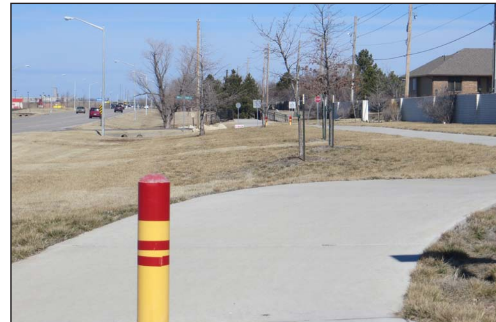
Shared-use paths offer cyclists a high degree of separation from vehicles, and are often used by cyclists of varied skill levels. Source: Parsons Brinckerhoff (existing shared-use path along S. Kansas Avenue, Newton, KS)
