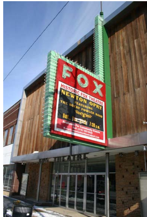
Above is an example of a unique projecting (or “blade”) sign that has attained historical significance in its own right. Such signage merits retention and preservation.
