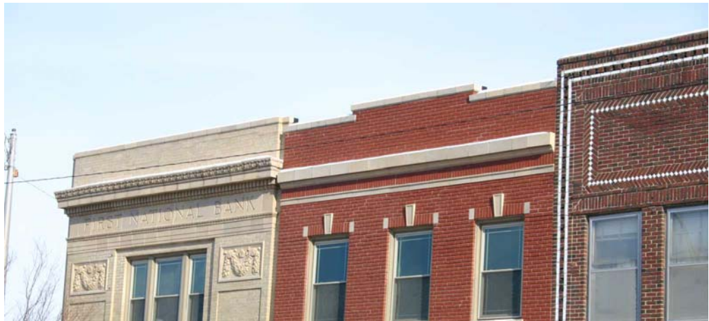
Stone, brick, and in some cases terra-cotta and cast iron are typical materials for downtown.
