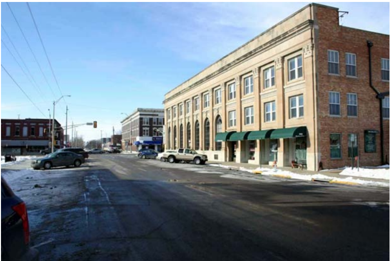
An excellent example of secondary facades and pedestrian-friendly entryways along East 5th Street.
