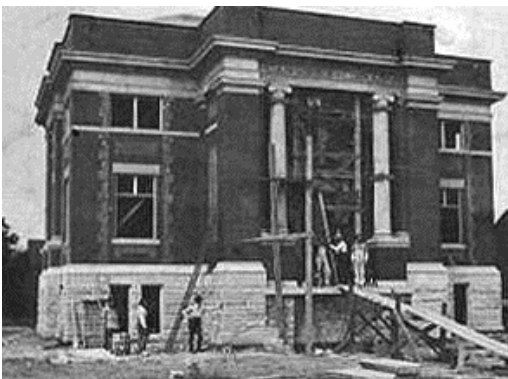
The Carnegie Library under construction, 1903.
