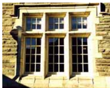
AFTER: Cleaned stonework and matching replacement windows after rehabilitation.
