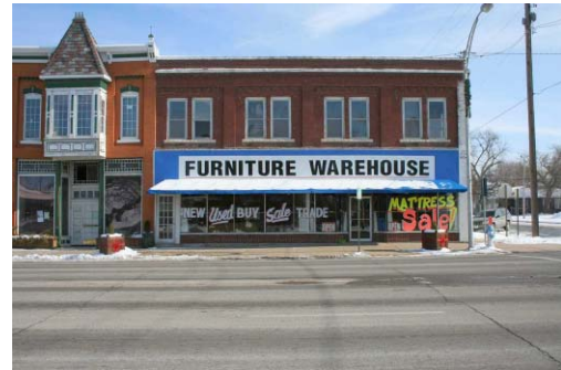
Historically significant buildings are important in defining the character of the district. The J. S. Dillon and Son's Grocery building has provided retail services at street level since 1909.
