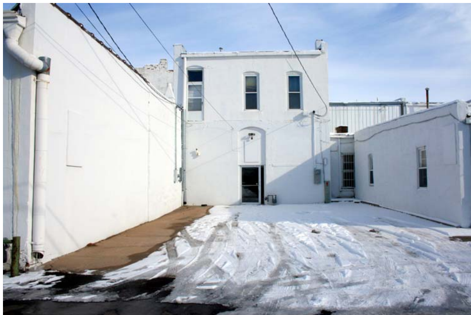
Secondary and rear facades should retain their patterns of window and door openings.
