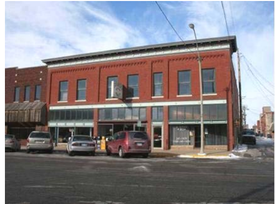
A ribbon of historic transom windows defines the break between the street-level commercial uses and upper-story functions for this historic building.
