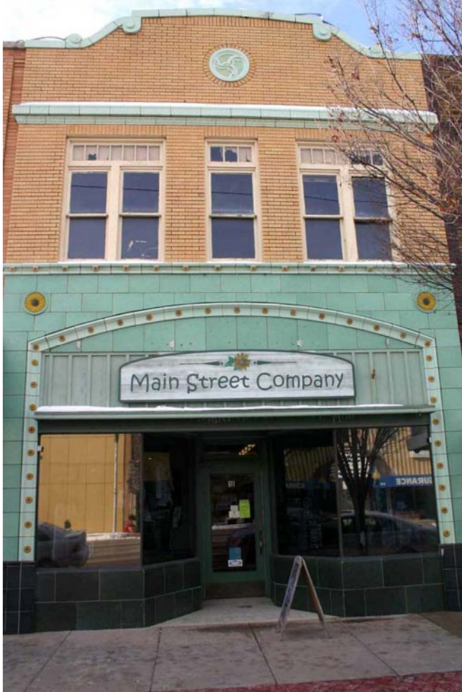
The facade at 611 North Main provides an excellent example of how brick, stone, wood, glass, and terra-cotta materials may be combined to create an effect of high visual interest.
