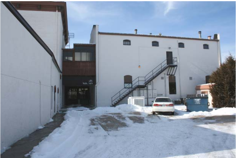
Rear and secondary entryways may be architecturally interesting but should not compete with the primary facades of buildings.
