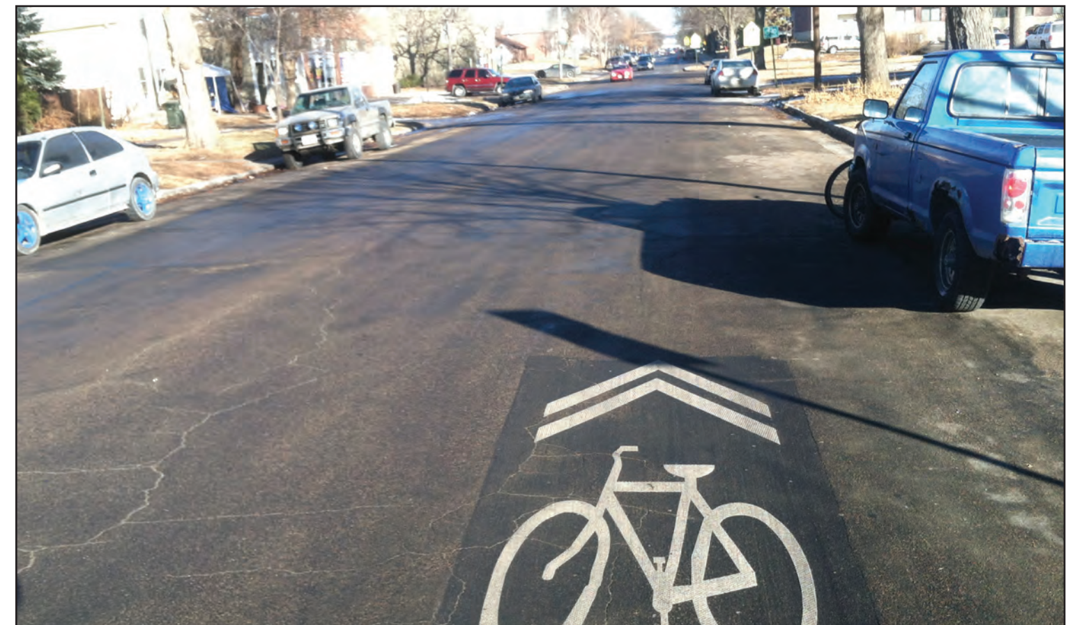
Shared-Use Markings help cyclists safely position themselves to the right of traffic but left of the area where doors of parked cars open. Source: Parsons Brinckerhoff (Lincoln, NE)
