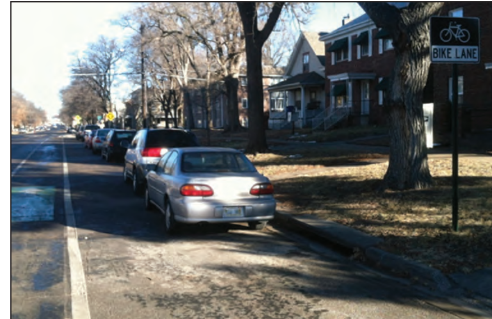
This bicycle lane design in Lincoln, Nebraska took advantage of the existing wide width of the street to give motorists ample space to park and swing open doors. Source: Parsons Brinckerhoff (Lincoln, NE)
