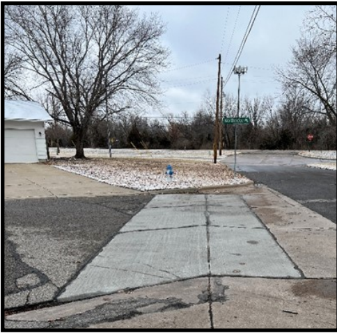
Gutters were replaced at Northridge Road and Terrace Drive (left) and 5th Street and Columbus Avenue (right) to improve drainage
