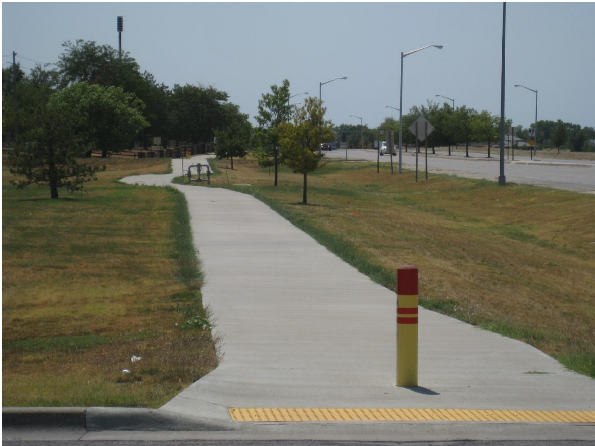
Figure 7 - Shared-Use Path on the East side of South Kansas Avenue (12 th Street to SE 24 th Street) Source: Parsons Brinckerhoff
