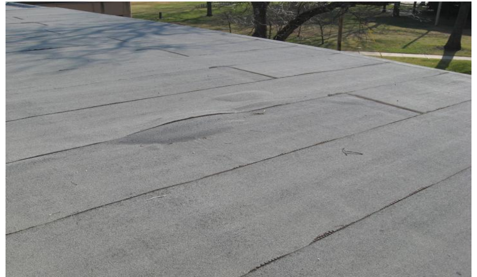
PHOTO 24 BUBBLED ROOFING
