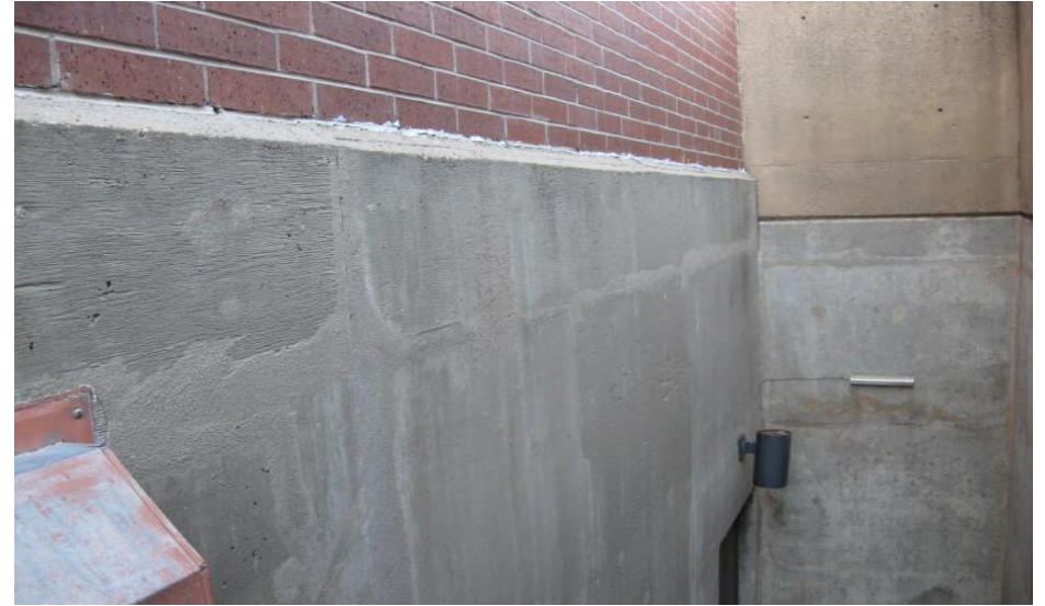
PHOTO 6 NORTH AREAWAY CONSTRUCTION JOINT AT DOUBLE TEE BEARING
