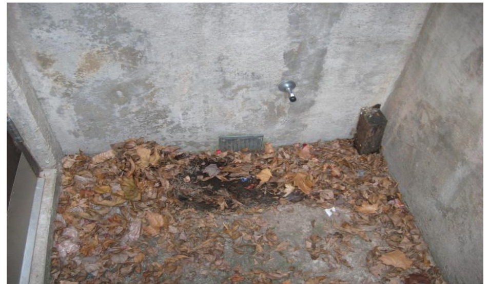
PHOTO 20 BOTTOM OF AREAWAY - POTENTIAL FOR BLOCKED DRAIN
