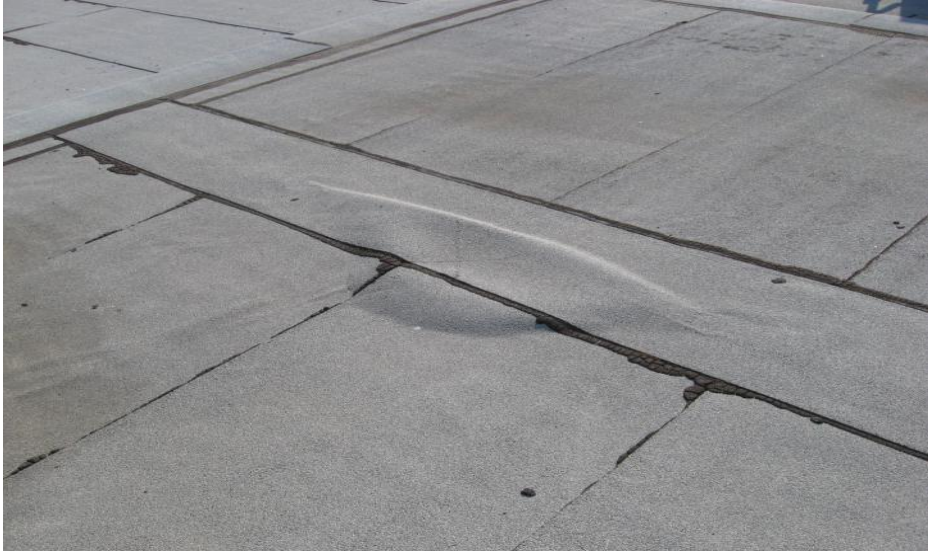
PHOTO 25 BUBBLED ROOFING
