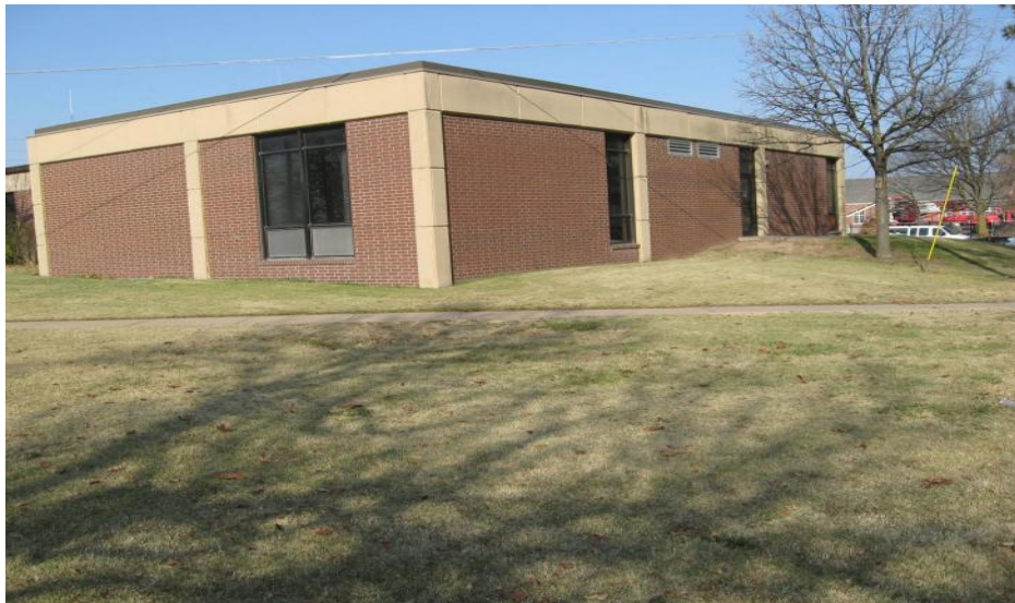
PHOTO 43 SITE GRADING AT SOUTHEAST BUILDING CORNER
