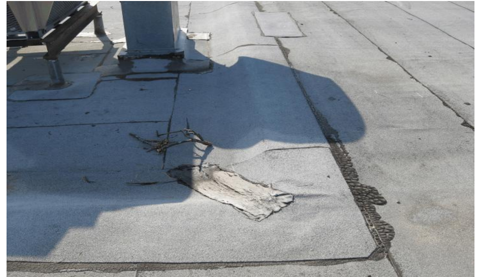
PHOTO 48 ROOF TRANSITION BETWEEN ORIGINAL BUILDING AND BUILDING ADDITION
