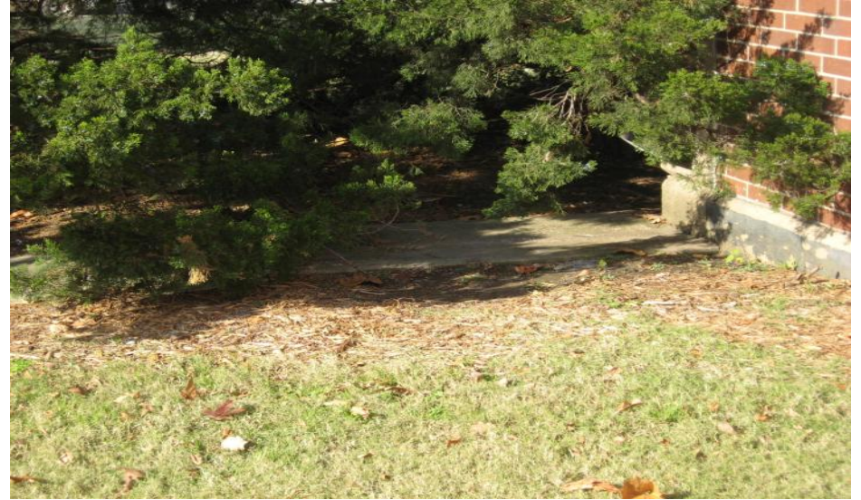
PHOTO 22 SPLASH BLOCK DRAINS TO BUILDING
