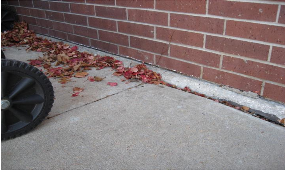
PHOTO 9 OPEN SLAB JOINT - RAKED MASONRY BED JOINT
