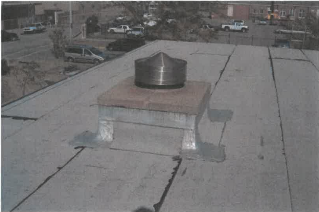
4.1.1.4. – Boiler Flue – View 1921
