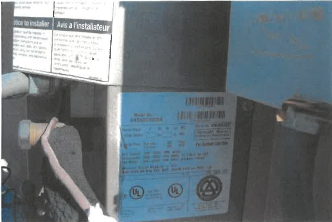
4.1.1.6.1.2. Deteriorated Pipe Insulation – Unit #2 – View 1909
